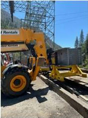
^Moving Spreader Beam
