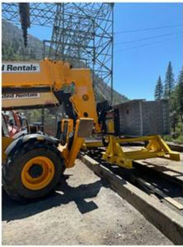
^Moving Spreader Beam
