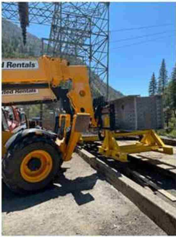
^Moving Spreader Beam
