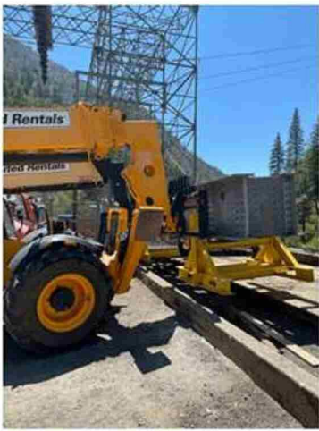
^Moving Spreader Beam
