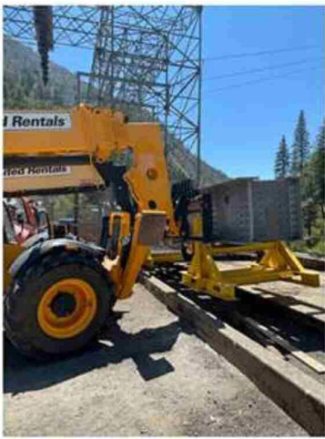
^Moving Spreader Beam
