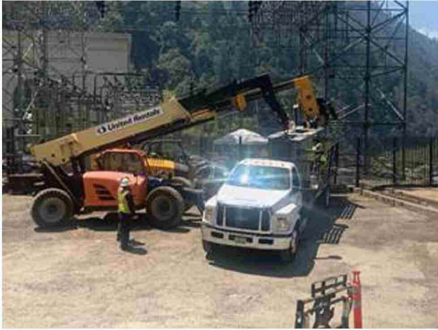
^Relocating Spreader Beam to Powerhouse
