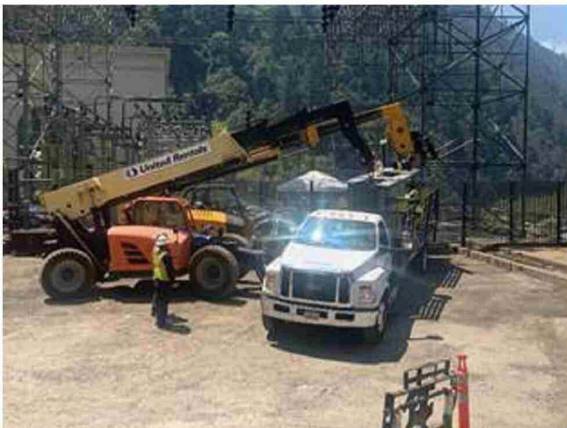
^Relocating Spreader Beam to Powerhouse
