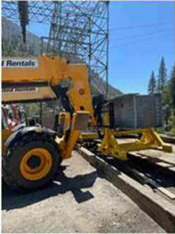
^Moving Spreader Beam
