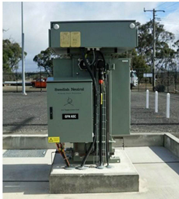
FIGURE PG&E-7.3.3-5: ARC SUPPRESSION COIL / GFN
